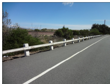
Historic timber guard-rail
