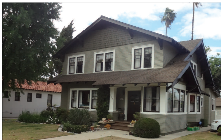
1164 E. Grand Blvd after painting is completed
