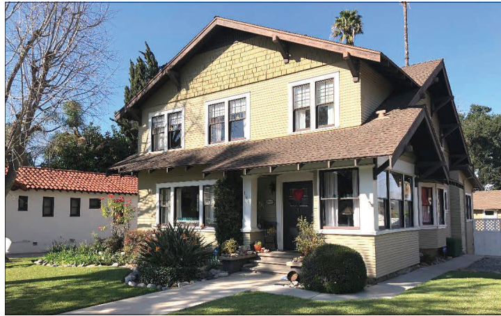
1164 E. Grand Blvd before repainting
