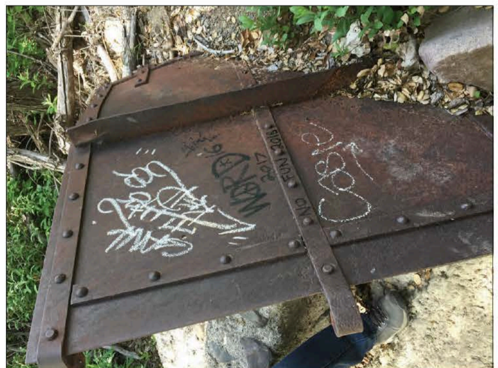
Abandoned sluice gate located in Hagador Canyon
