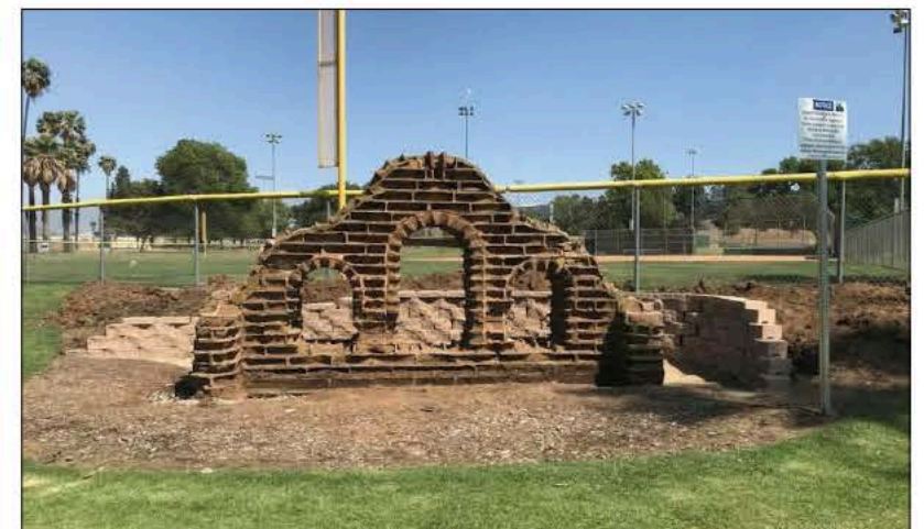
Appearance of the wall awaiting restoration work
