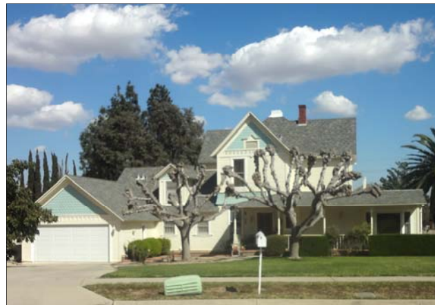
This image, with the address of 1441 Beechnut Lane, shows what was once the rear elevation of the home.
