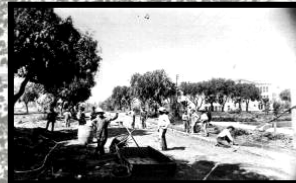
Laying down sidewalks and curbs, 1911.
